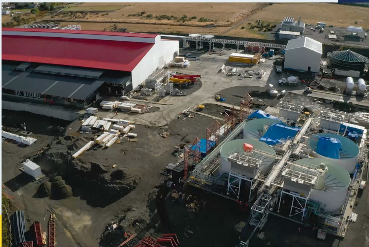
Dumestre Hydrobiological Resources Processing Plant (Chile) – CICDHA. © Greenpeace
