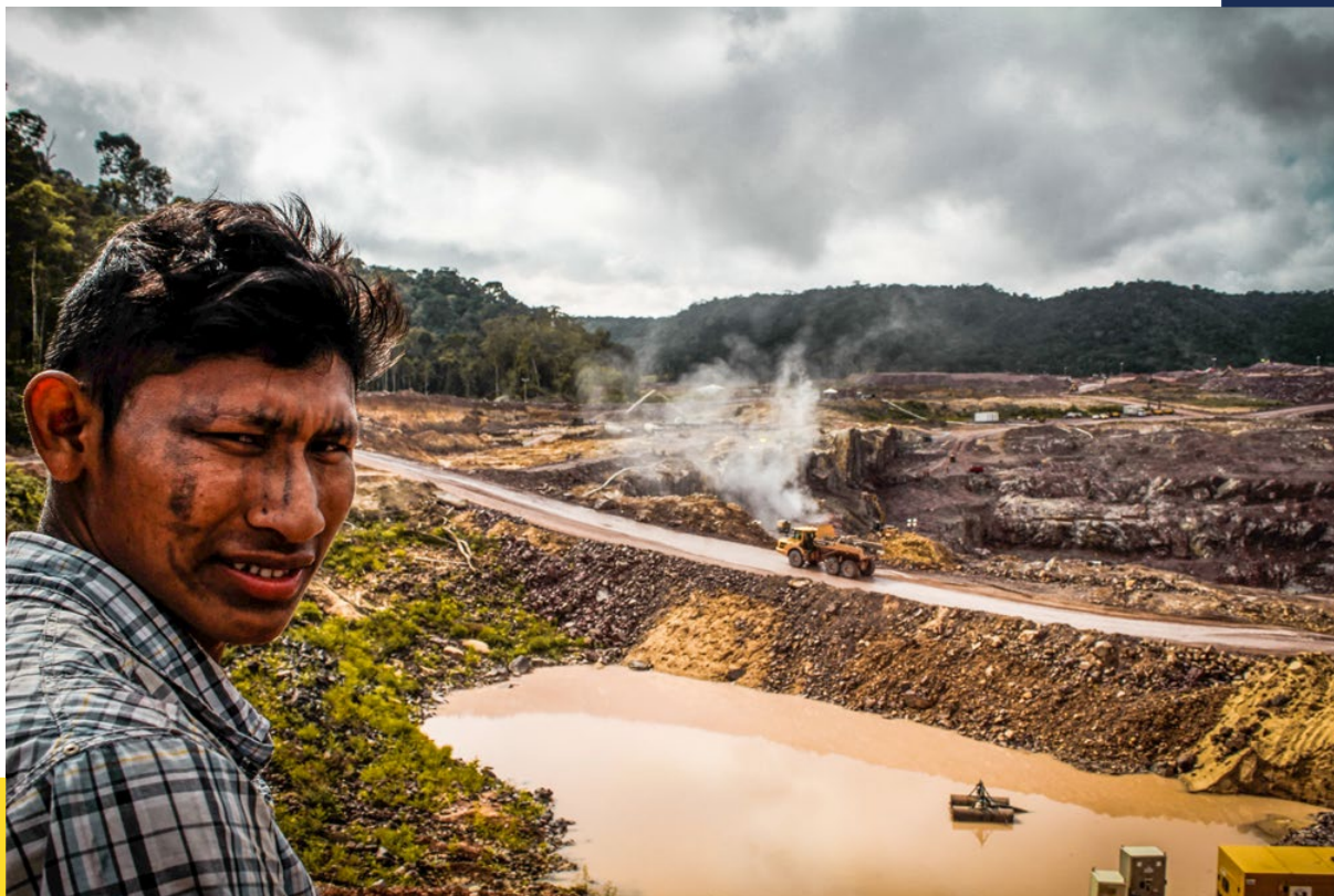
Kayabi leader observing the start of construction of the São Manoel hydroelectric plant in his territory. © Caio Mota, Coletivo Proteja
