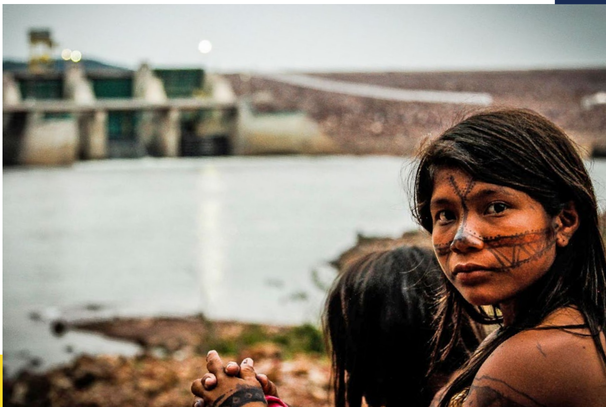
Child of the Mundurucu people observing the destruction caused by the São Manoel hydroelectric power plant in their territory. (Brazil) © Juliana Pesqueira, Coletivo Proteja, 2017
